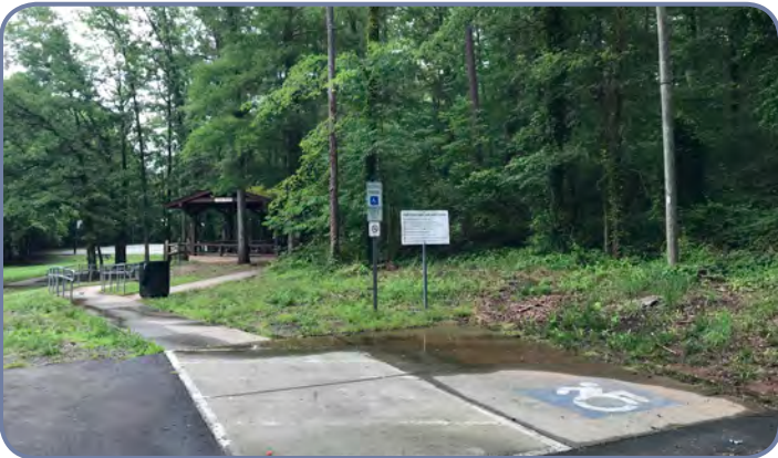
Stormwater ponding and hillside washout impact the usability of the ADA parking space.
