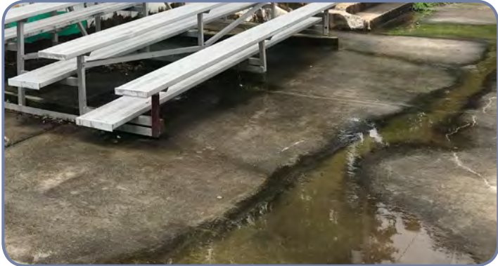
Stormwater is ponding and creating very slick conditions near the baseball field.
