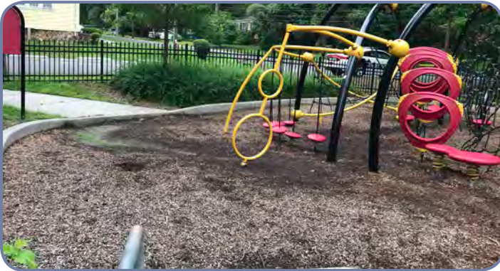
The playground surface is washing down the hill and the engineered wood fiber (EWF) surfacing can be seen on the ADA pathway down toward the swings.
