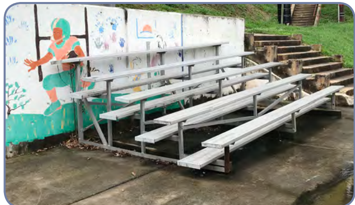
The bleachers for the baseball field appear disheveled or broken. The stone steps in the background are in disrepair and lack a railing.
