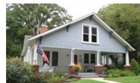
Attached: 1212 Vickers Avenue
