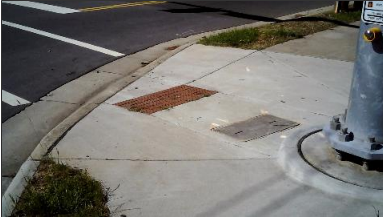
Acceptable Texture and Color Contrast Curb Ramp
