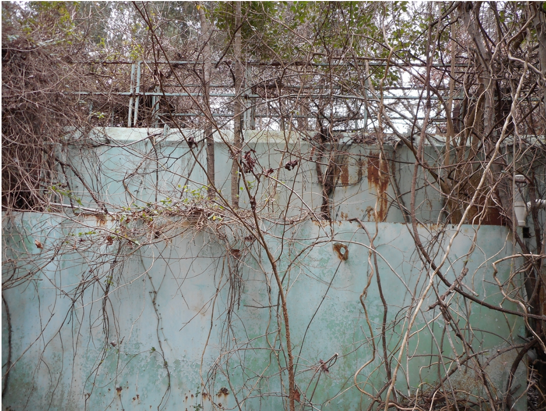
Photo 7: Tank to be demolished at Farrington Rd. WWTF
