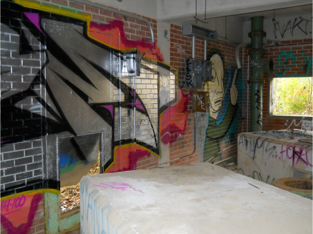
Photo 2: Interior of 2-story building at Hope Valley WWTF
