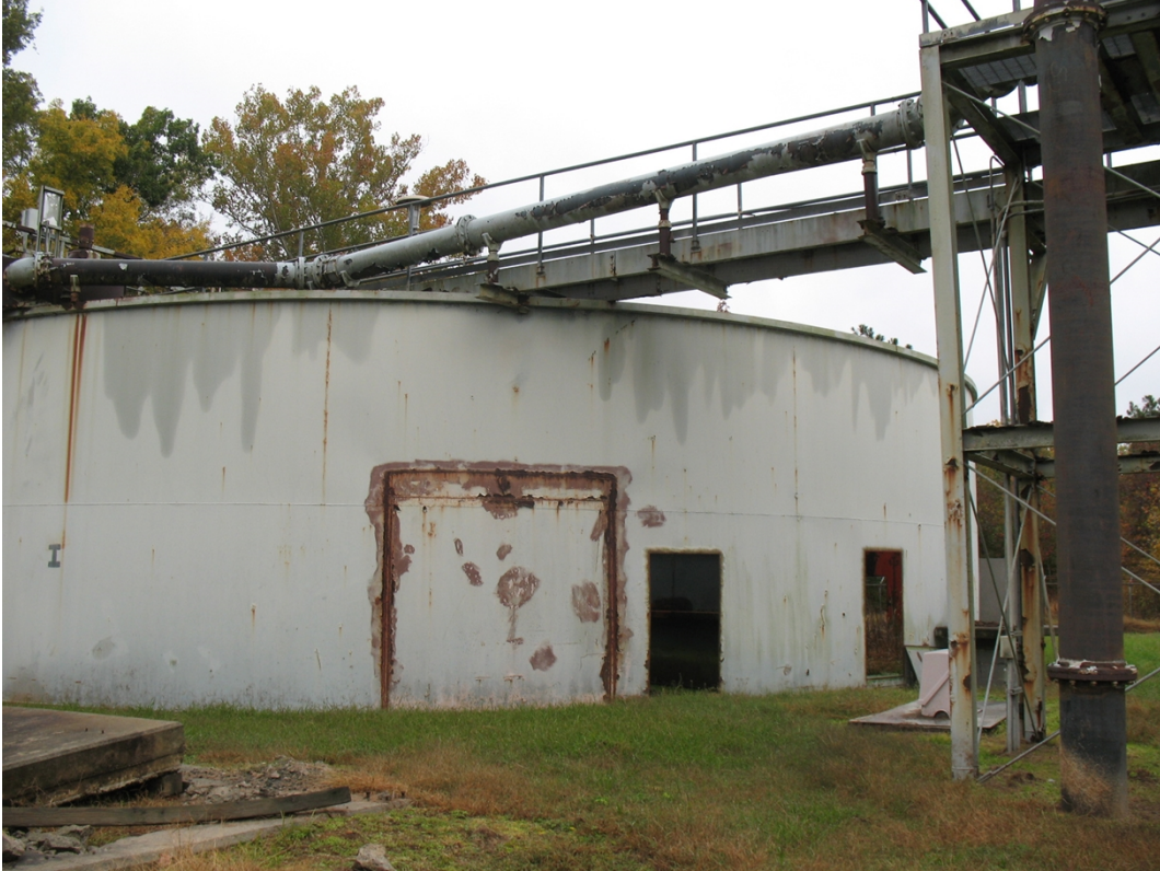
Photo 9: Tank 1 to be demolished at Eno WWTF
