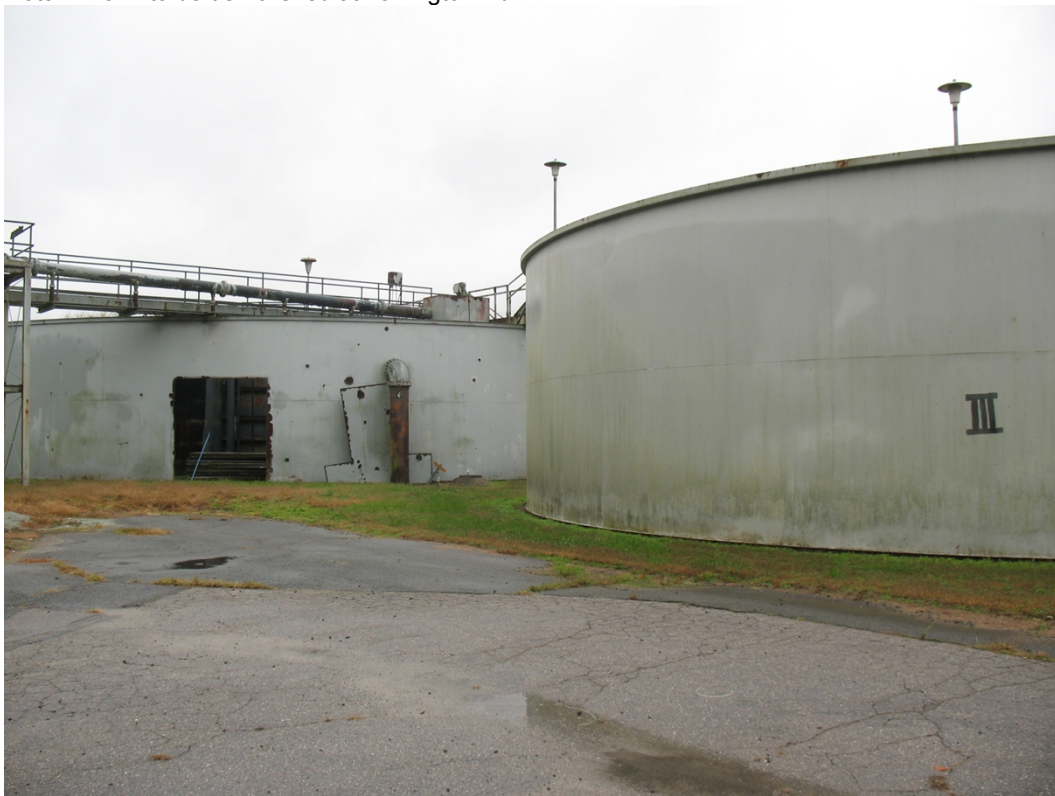
Photo 8: Tanks 2 and 3 to be demolished at Eno WWTF
