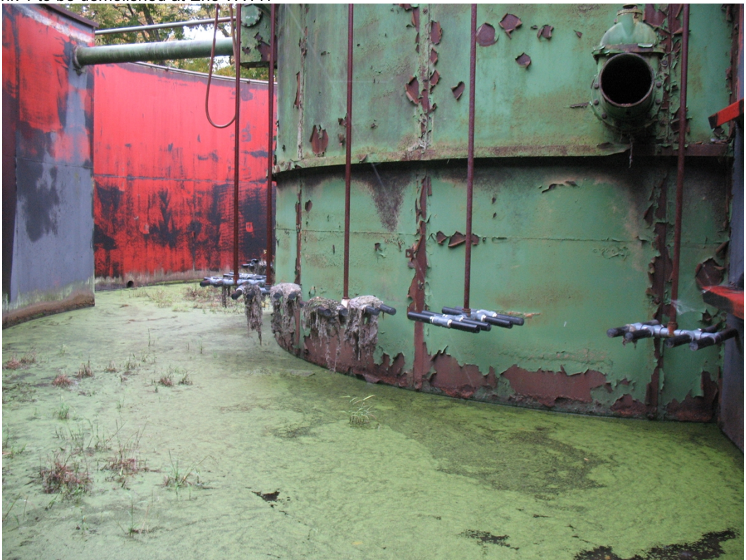
Photo 10: interior of tank to be demolished at Eno WWTF
