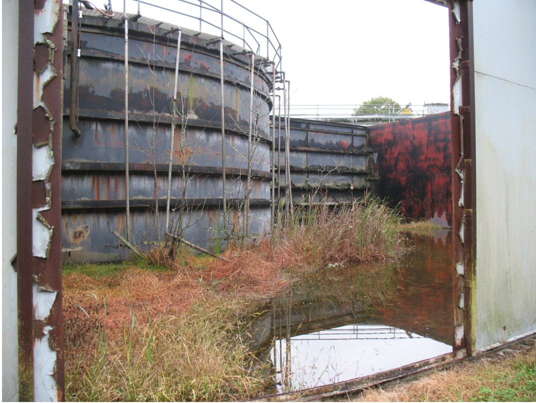
Photo 11: Interior of tank to be demolished at Eno WWTF
