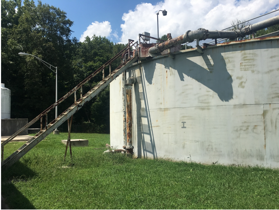
Photo 13: Tank to be demolished at Lick Creek WWTF
